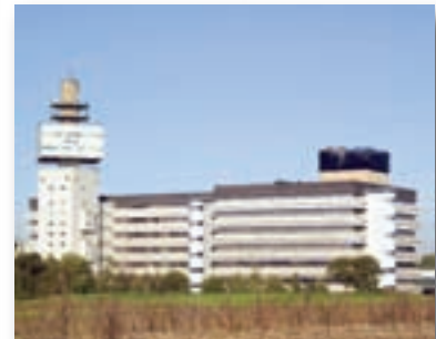
Bronze reflective film applied to BT Laboratory Buildings
