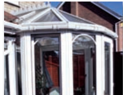
Conservatory with solar control film applied
