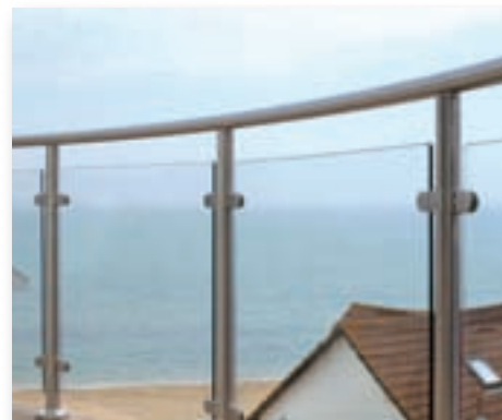
Glass balustrade at a residential development in Norfolk
