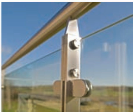
Balustrade fixings using both pig nose bolts and glass clamps
