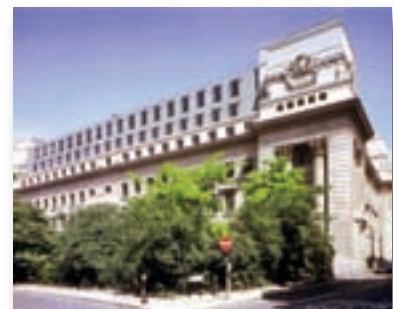
Combined solar/safety film applied to Grade II listed building
