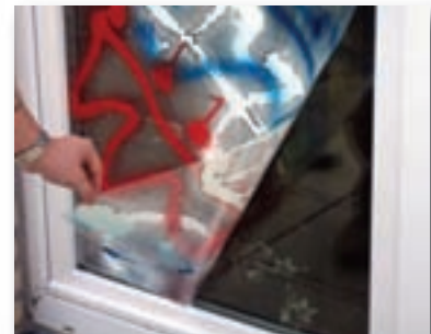
Anti-graffiti film being removed
