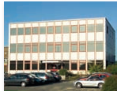
Silver reflective film applied to Suffolk Fire Service HQ
